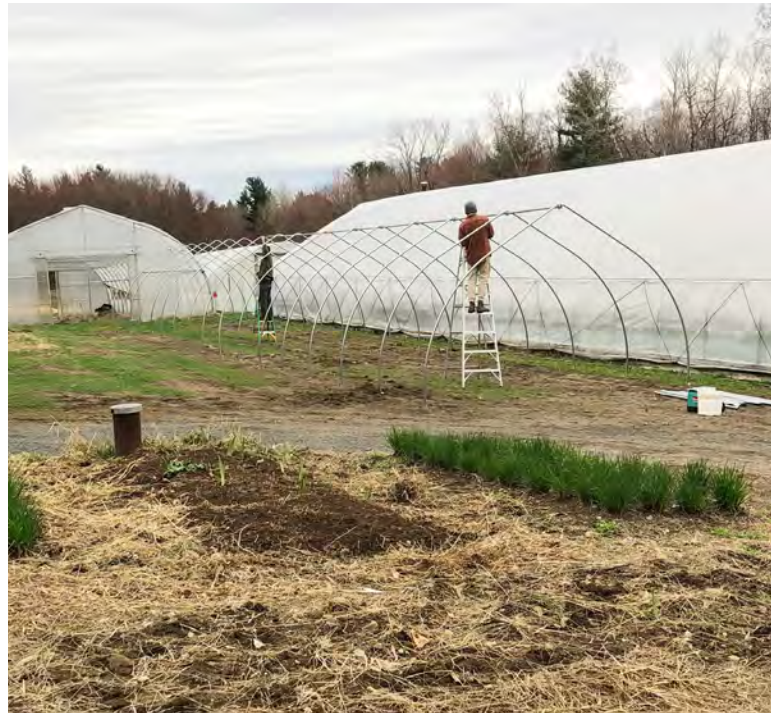
Ellen and Ben construct our new moveable cold frame
